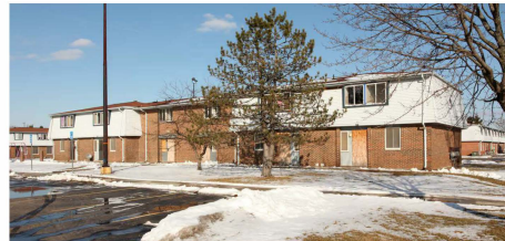
Continue Facade Improvements at River Park
